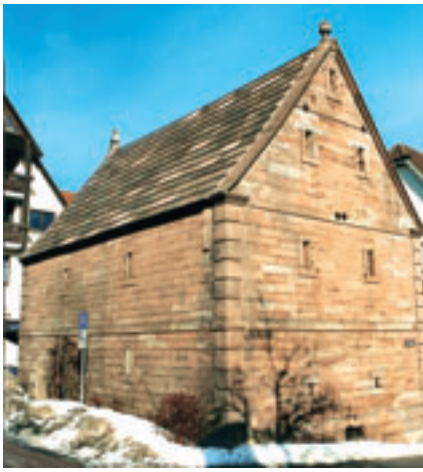
Loßburg, Alter Speicher.
